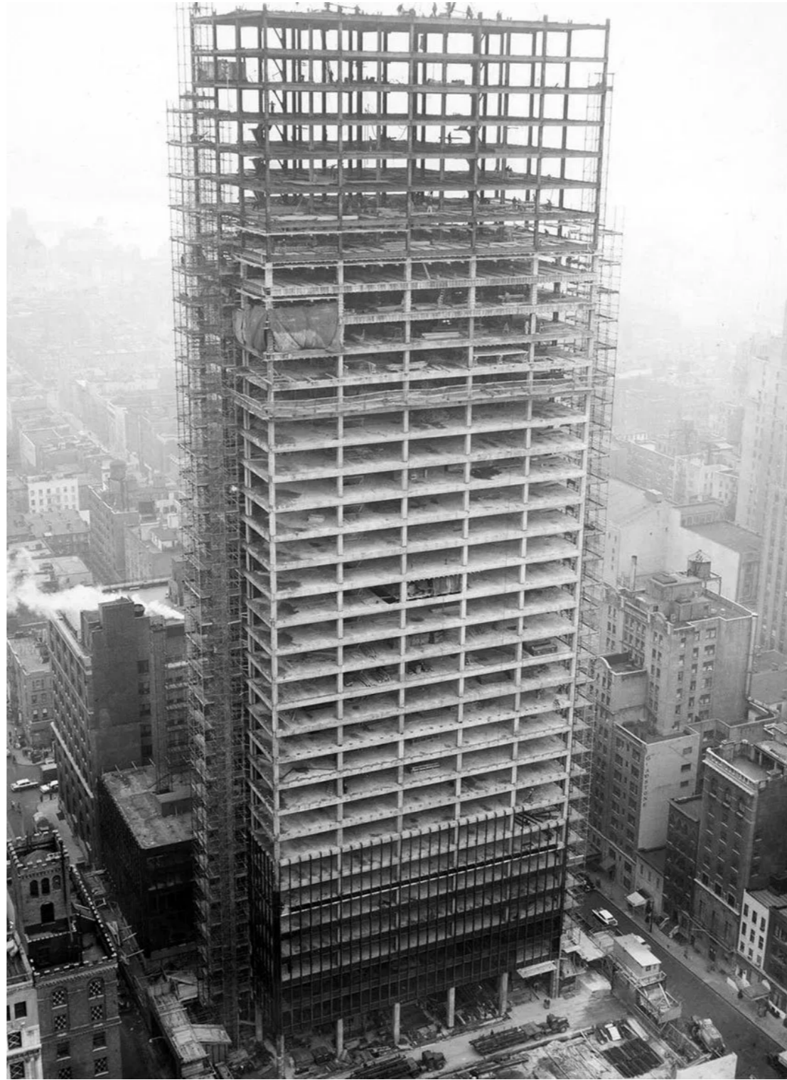
Seagram Building construction , NYC, Mies van der Rohe, 1958
