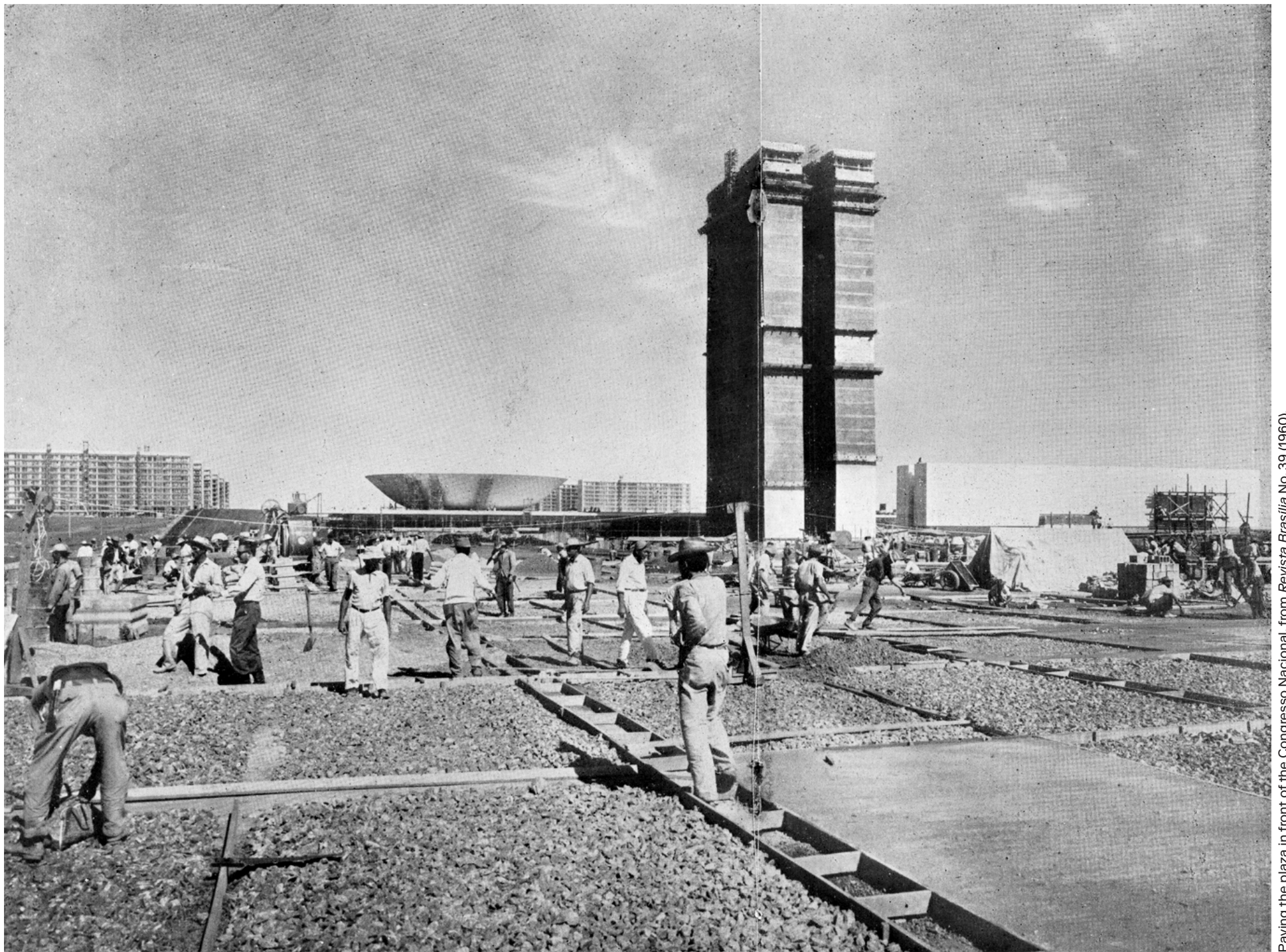
Paving the plaza in front of the Congresso Nacional, from Revista Brasília No. 39 (1960).
