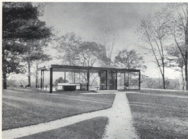
Philip Johnson, Philip Johnson House , New Canaan, Connecticut, 1949.
